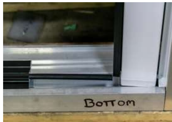
Extend track runner, lift pull bar
