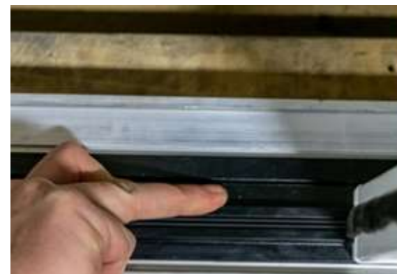
Interlock the track and fit in retaining spline
