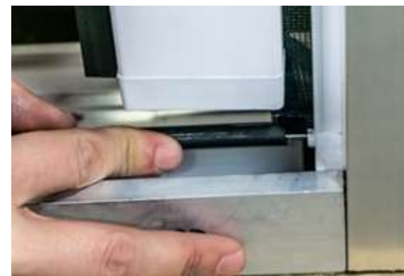
Slide over metal guide onto mesh, tight to housing nipple
