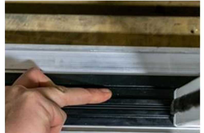
Interlock the track and fit in retaining spline
