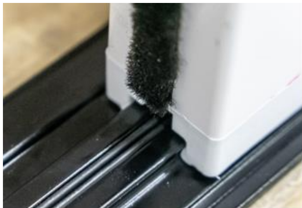
Feed lower track onto pull bar
