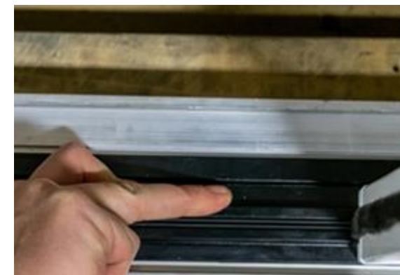
Interlock the track and fit in retaining spline
