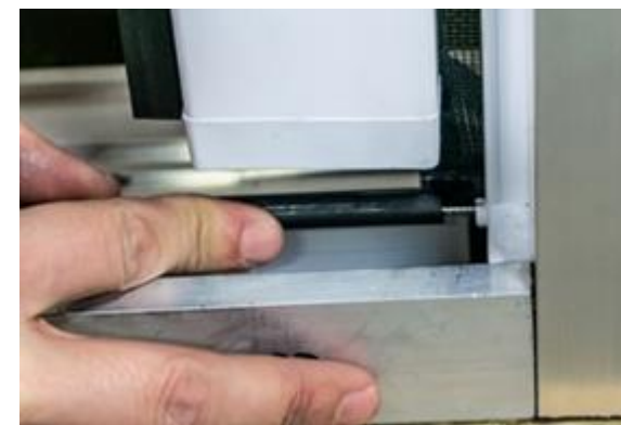
Slide track runner onto mesh, tight to each housing nipple
