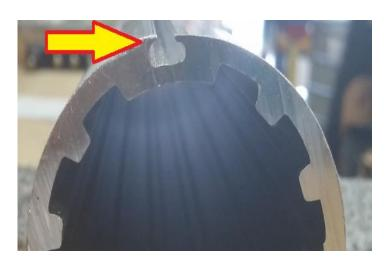
\*Tip – Unroll existing mesh and line up new mesh the same way onto roller tube
