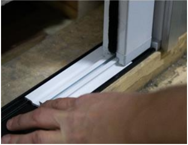
1. Remove track cut-off.
