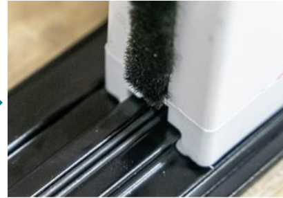
3. Feed lower track through pullbar.
