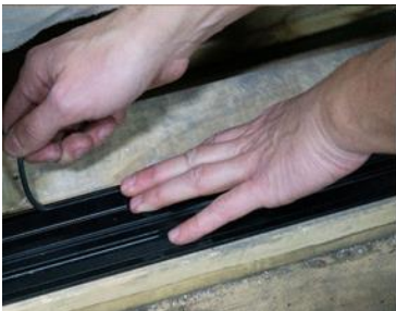
5. Interlock track and insert spline into groove.
