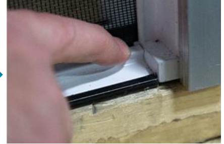
4. Push fully against housing – no gaps.
