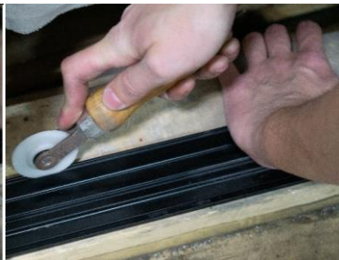
5. Interlock track and insert spline into groove.
