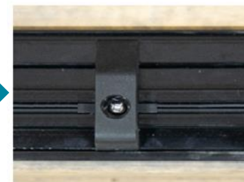
6. Attach lower track joiner
