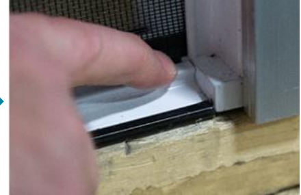
4. Push fully against housing – no gaps.
