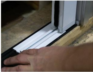
1. Remove track cut-off.
