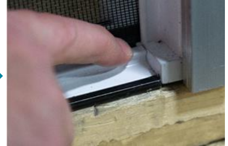
4. Push fully against housing – no gaps.
