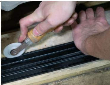
5. Interlock track and insert spline into groove.
