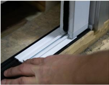
1. Remove track cut-off.
