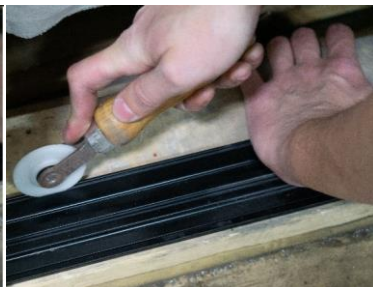
5. Interlock track and insert spline into groove.
