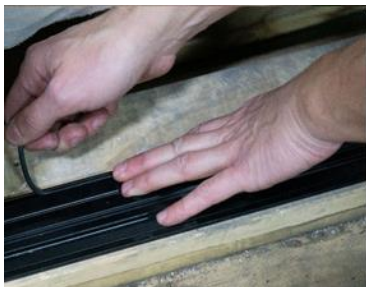
5. Interlock track and insert spline into groove.
