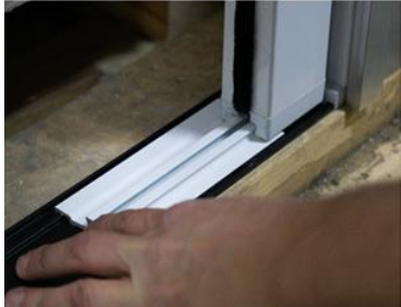
1. Remove track cut-off.
