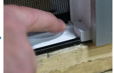
4. Push fully against housing – no gaps.
