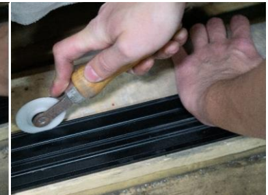
6. Interlock track and insert spline into groove.
