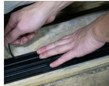
6. Interlock track and insert spline into groove.
