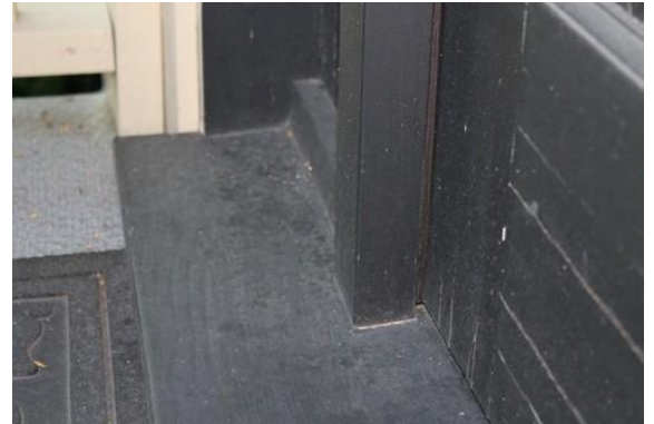
Threshold extends past moulding
