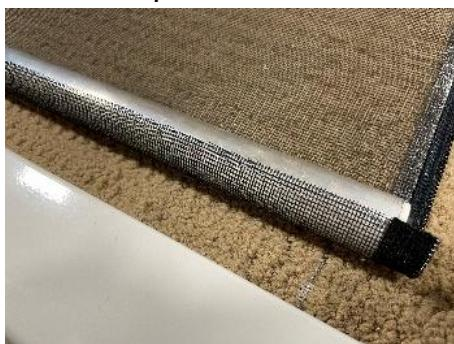
h) Apply **3M vinyl tape** over mesh and roll-tube evenly.
