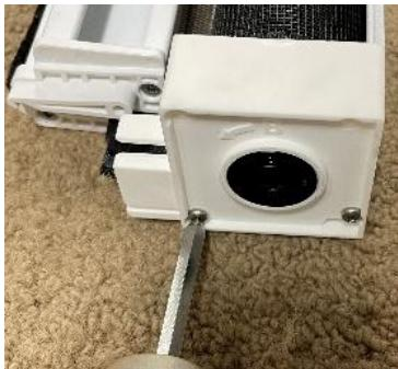
d) Reduce torque to **2** and screw **tensioner** to **speed reducer**, ensuring **tensioner** remains **flush** with **bottom of endcap**. **\*DO NOT OVER TORQUE!**
